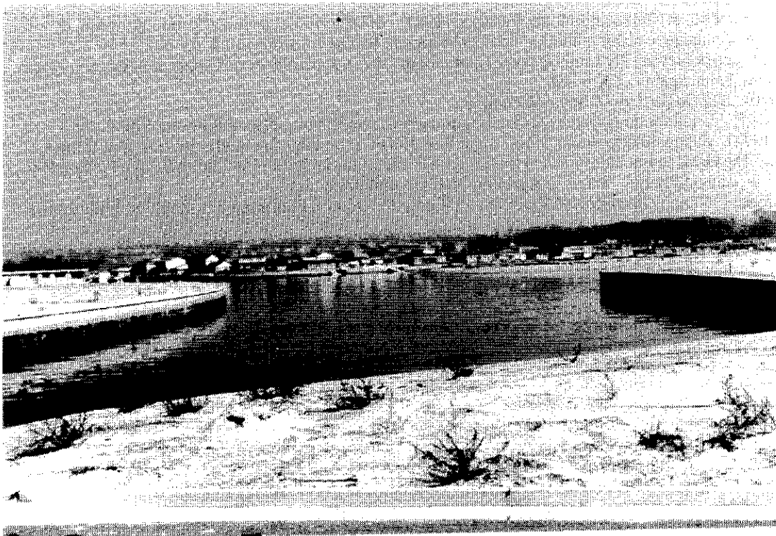
Sylvania Waters, Gawley Bay, Georges River, 1968. The first canal type development in New South Wales. Note vertical walls.
